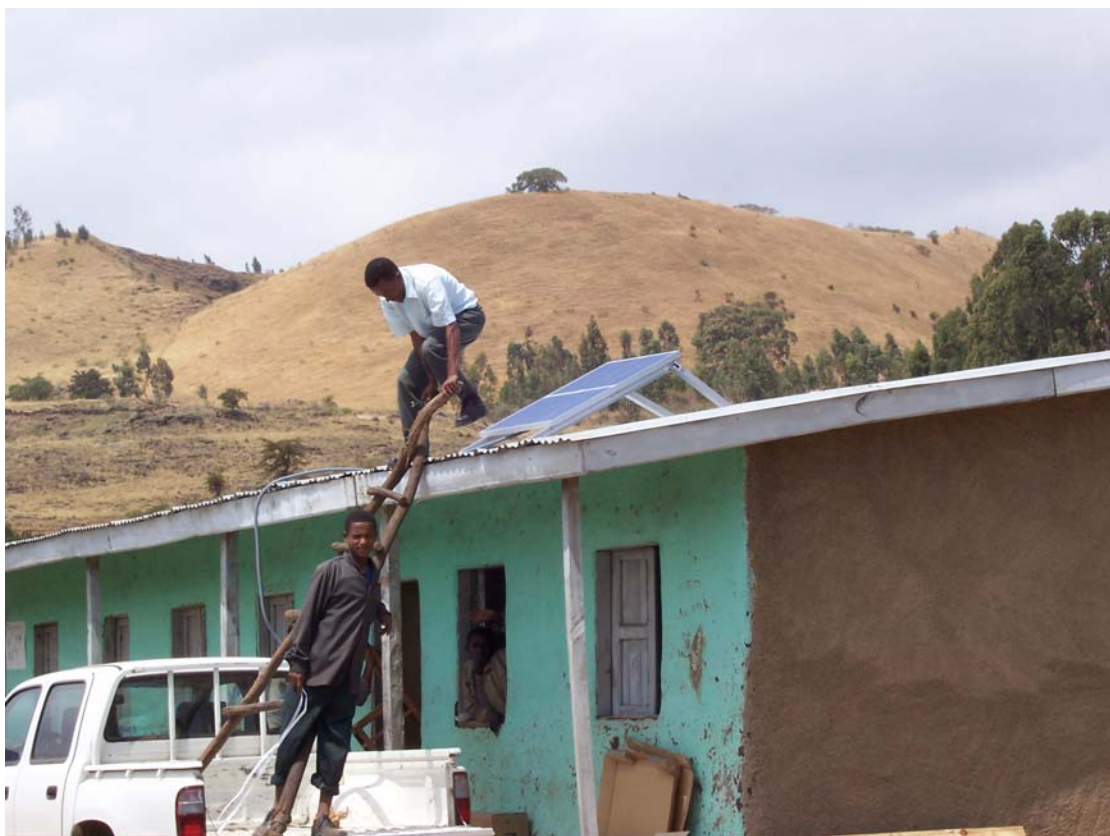
Plate 1: Solar panel installation in Dobotuto, Gurage
